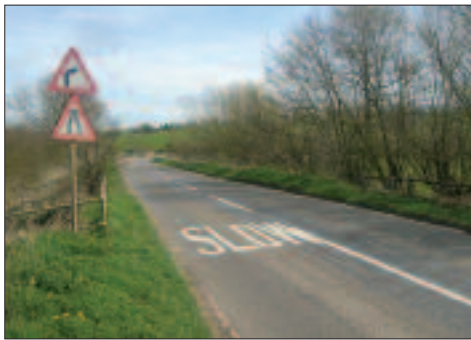
Approaching bridge from Spratton
